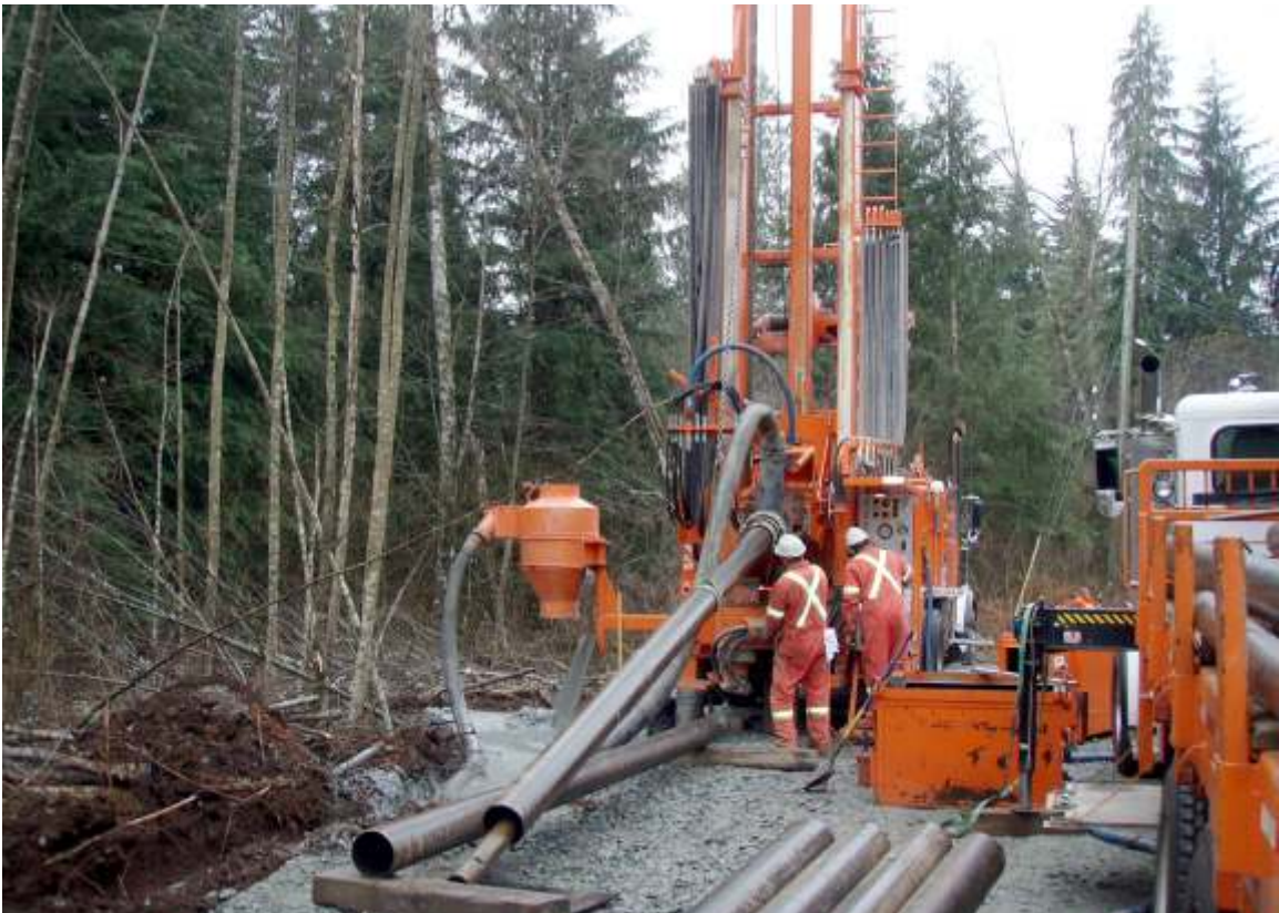
Photo 8. Drilling TW11-1 on December 6, 2011, with 20ft lengths of 8 inch well casing in foreground.
