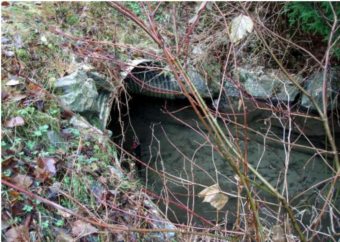
Photo 14. Durieu Creek gauging station at Durieu Road, December 6, 2011. Stilling tube is at outlet of culvert.
