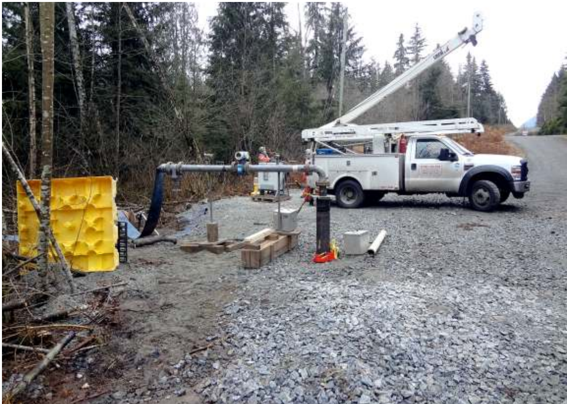
Photo 12. Equipment configuration at well head during pumping tests with TW11-1, December 14, 2011.
