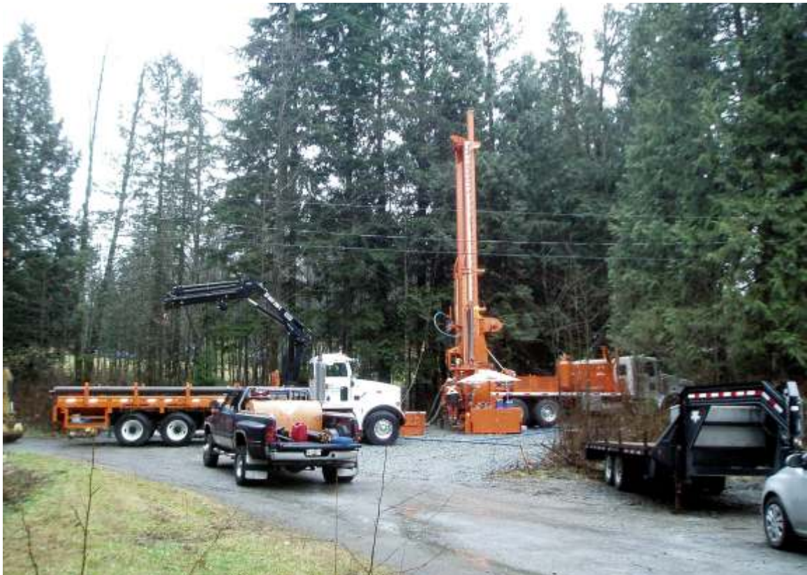
Photo 10. Drill rig and support truck at TW12-1, January 6, 2012.
