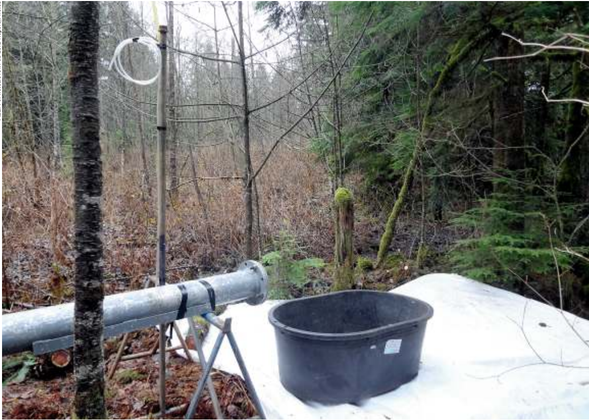
Photo 13. Orifice plate for measuring of well discharge rate during pumping tests with TW11-1, December 14, 2011.
