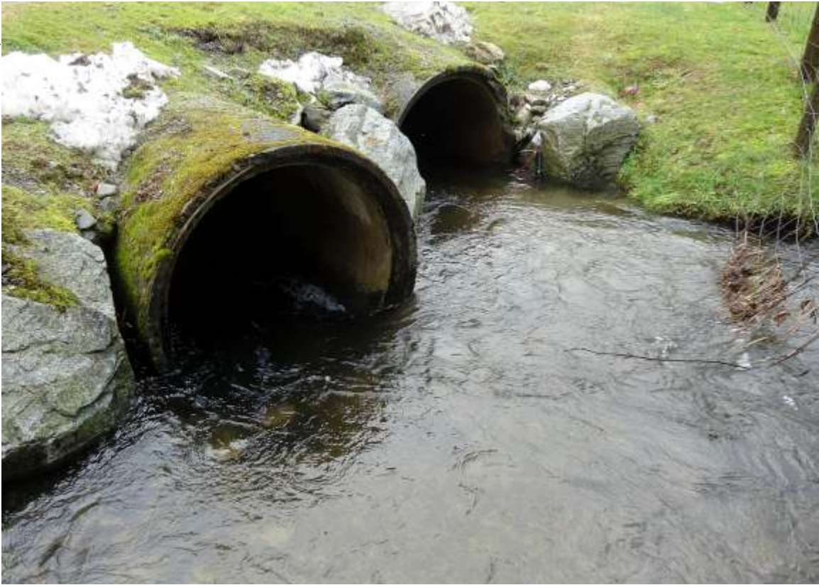
Photo 15. Oru Creek gauging station at Durieu Road, February 1, 2012. Stilling tube is at inlet of culvert in background.
